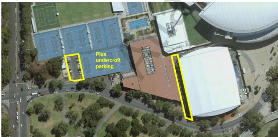
Figure 8: Permanent car parking permitted in Memorial Drive Tennis Club and Tennis SA leased areas
